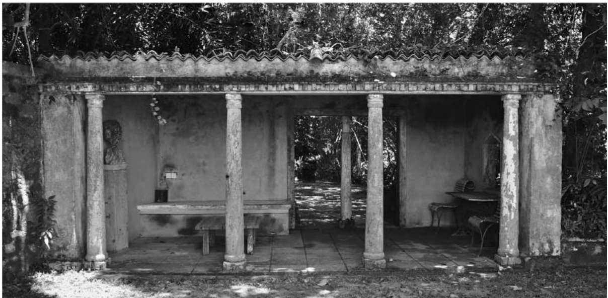
Figure 4. North View of the summer house garden. Photo by Jordan Wright.
