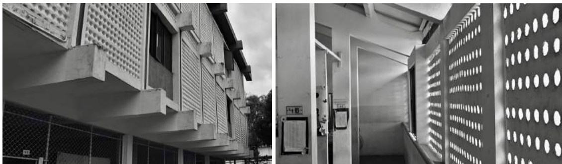
Figure 7. Classroom Block for Bishop's College, 2018, a view of the façade.
