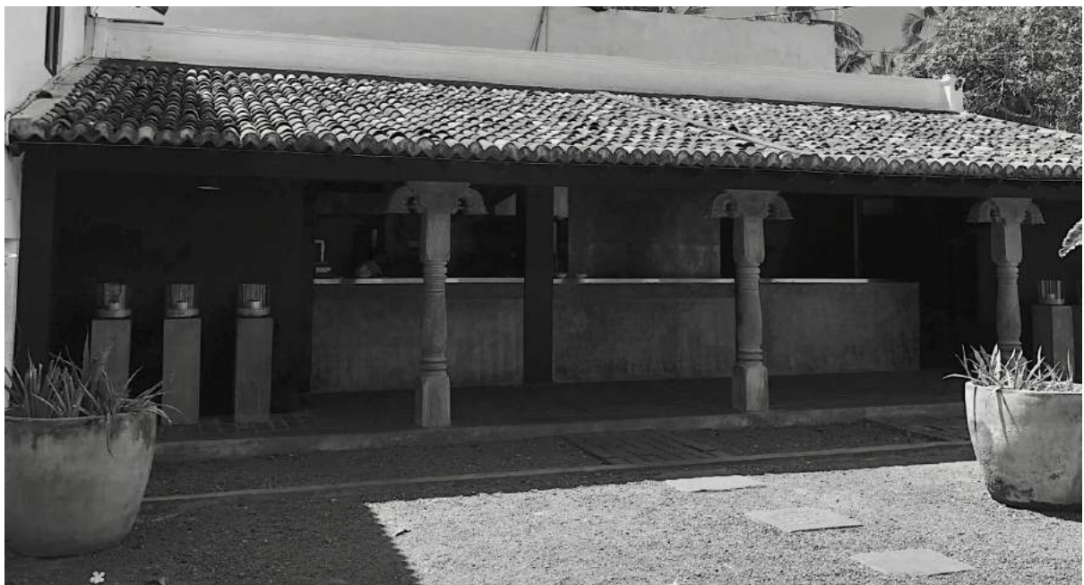
Figure 14. Walkway along the side of the building. Photo by Jordan Wright.
